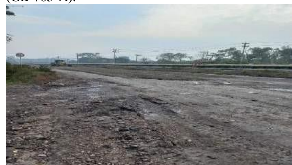
Figure 9. Grading activities of BP200 and BP60 materials on TS +35 - TLS 2 road
