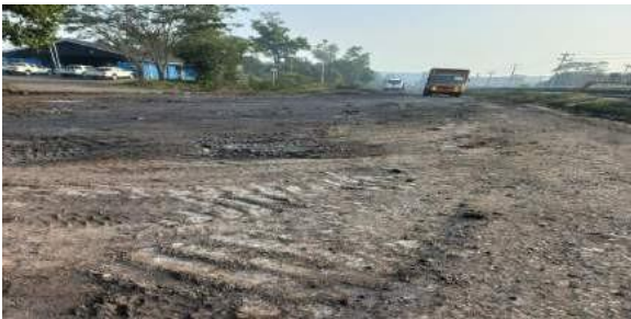
Figure 7. Condition of the road to be treated
