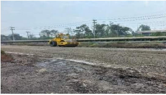
Figure 10. Road Compaction Activity
