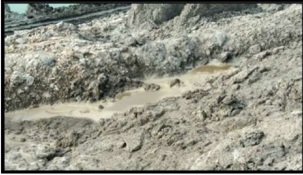
Gambar 2. Rembesan Air RL+40 mdpl Lereng Section A
