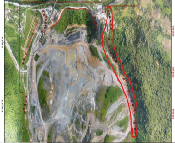
Gambar 7. Check Dam Tambang
