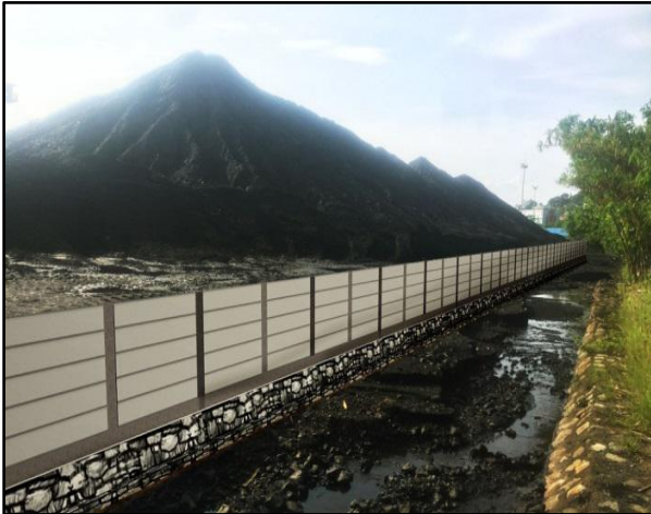
Gambar 18. Rancangan Dinding Penahan
