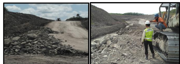
Gambar 18. Penambahan Ketebalan Base Coarse
