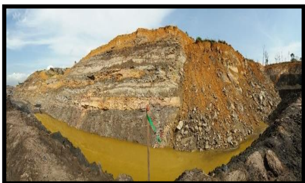
Gambar 9. Kondisi highwall Pit SB-II BK-14
