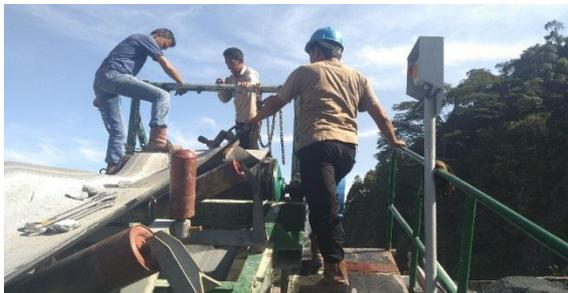
**Gambar 4.** Motor Pulley Rusak
