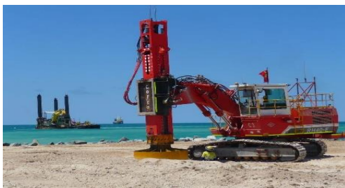
Gambar 1. Rapid Impact Compaction
