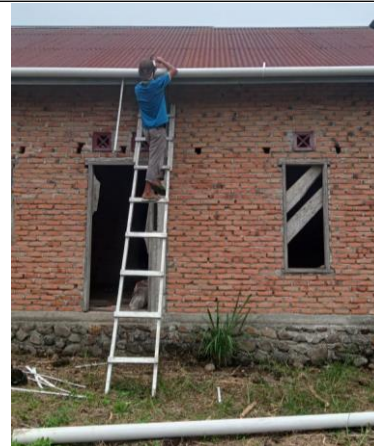
(f). Pemasangan talang air
