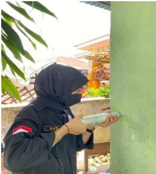
Gambar 3: Pengujian Hammer Test
